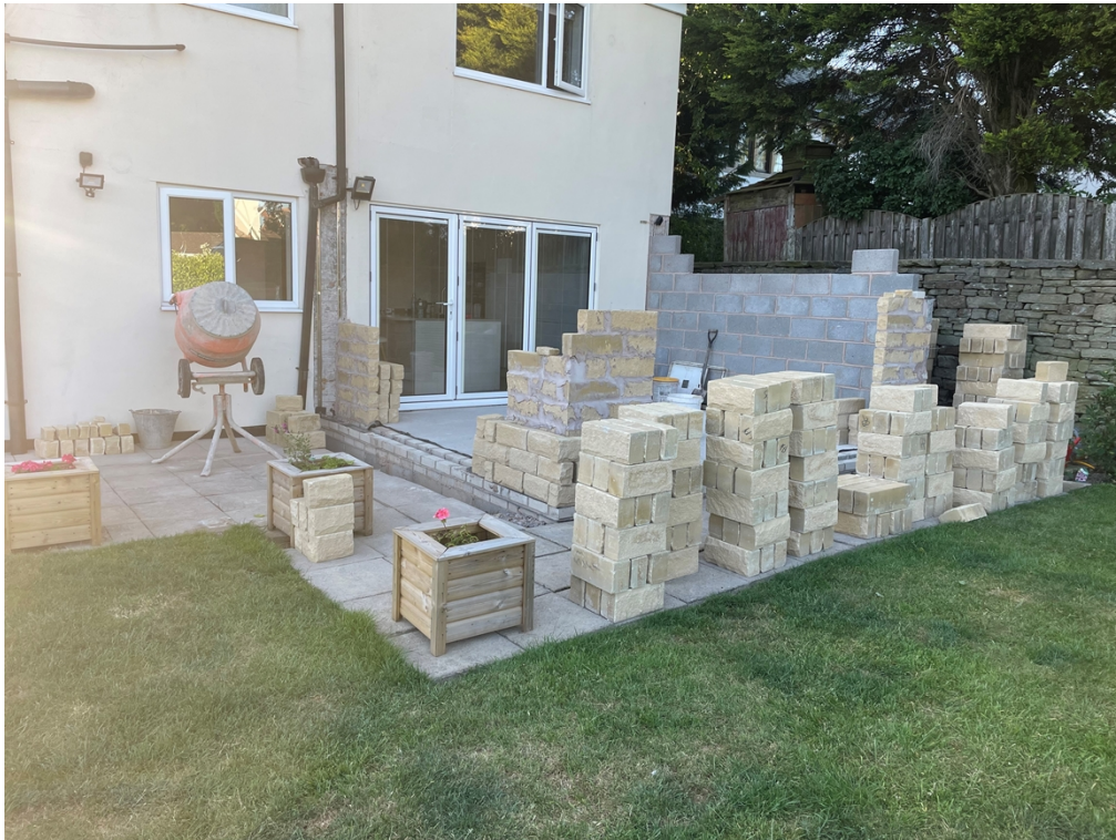
Extension under construction
